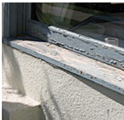
FIGURE 5.4a Peeling paint
