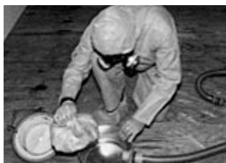
b) Disconnect Vacuum Bag From Hose Inlet
