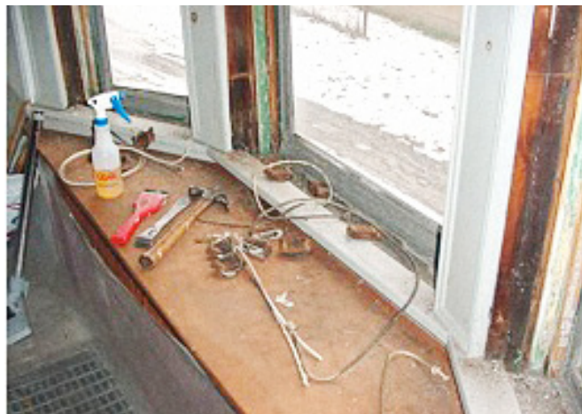
FIGURE 11.9 Window after removal of sash weights.
