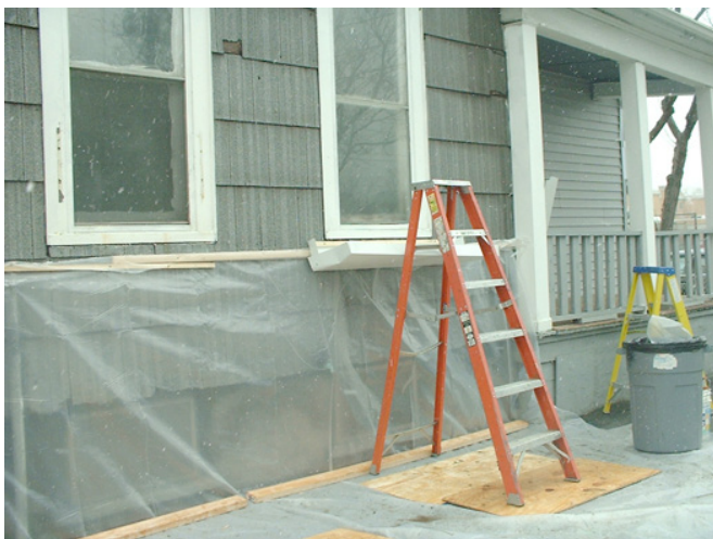
FIGURE 8.15 Exterior containment on building and window; ladder kept on plywood.
