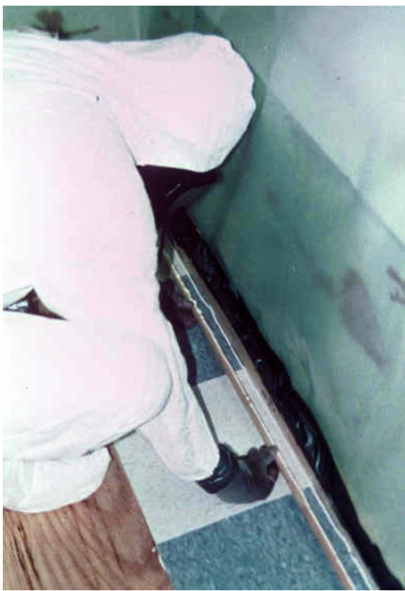
FIGURE 13.1 Encapsulating a floor with vinyl tiles
