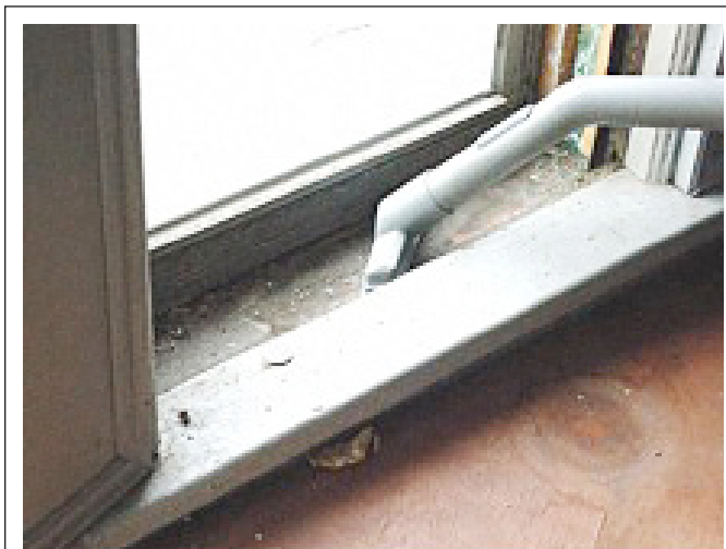
FIGURE 11.5 Prepare the worksite and pre-clean the window.
