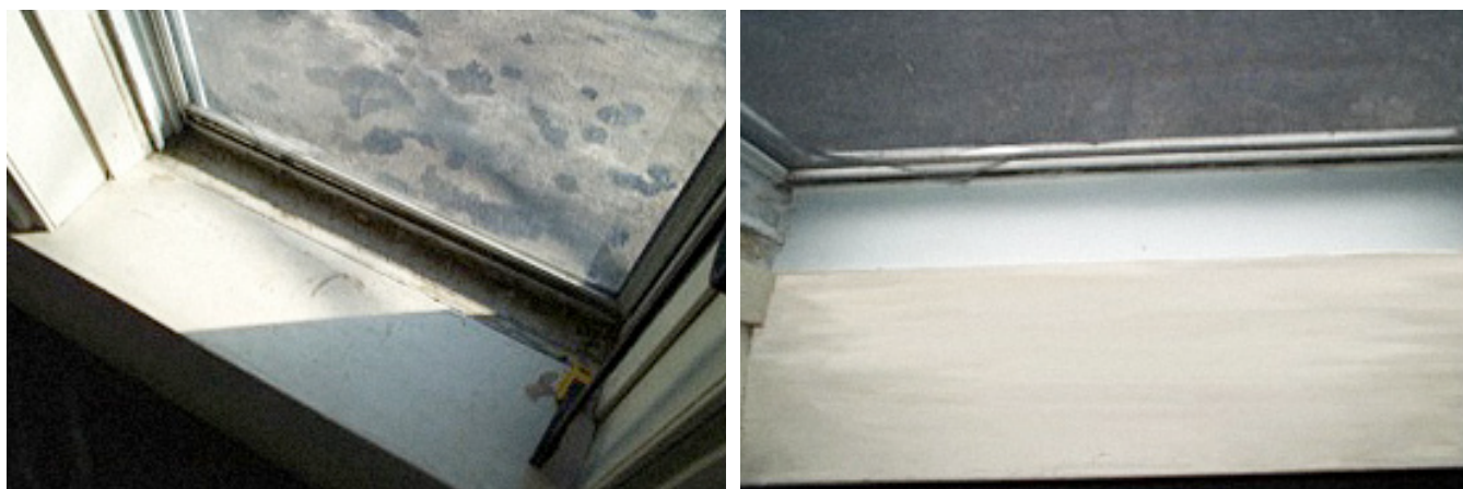
FIGURE 11.20 Turning a Window Sill and Trough Into a Smooth and Cleanable Surface. Window pre-treatment (left) and post-treatment (right).
