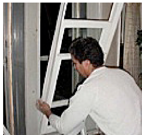
Figure 11.14 Reinstall sash into jamb.
