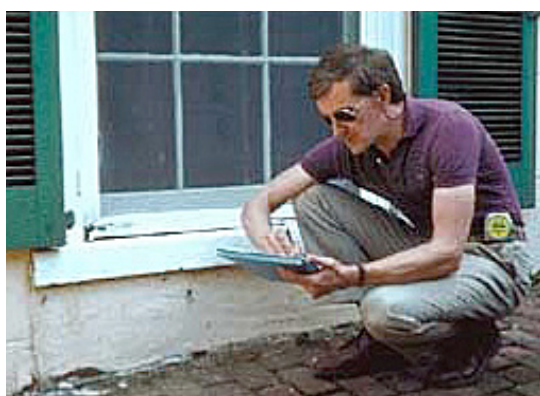
FIGURE 18.2 Historic properties should have a window condition assessment preceding work. Photo Courtesy National Park Service.
