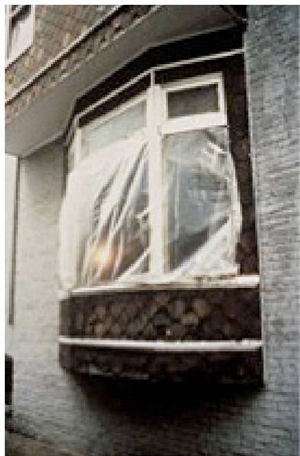
FIGURE 15.1 Windows sealed to prevent migration of dust outside.
