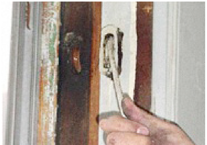
FIGURE 11.8 Remove sash controls/weights.
