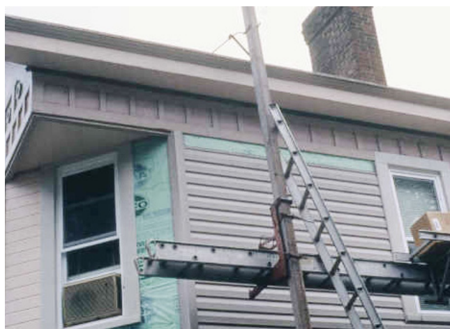
FIGURE 12.6 Installation of replacement siding.
