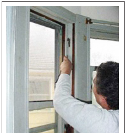
FIGURE 11.6 Remove parting Aboard.
