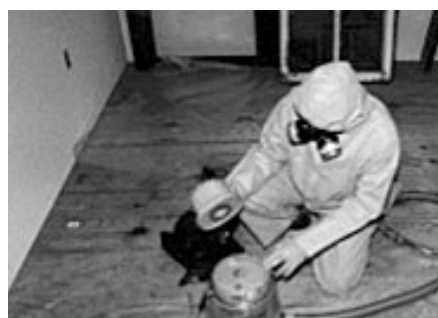
f) Remove & Replace HEPA Filter Assembly.
