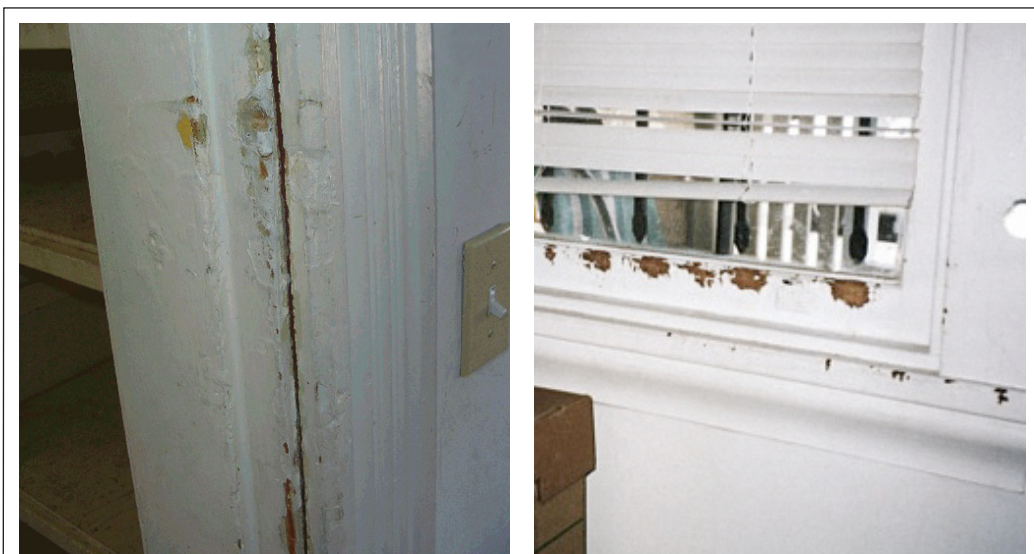
FIGURE 11.4 Examples of impact surfaces (left) and chewable surfaces (right). The window sash has large teeth marks.
