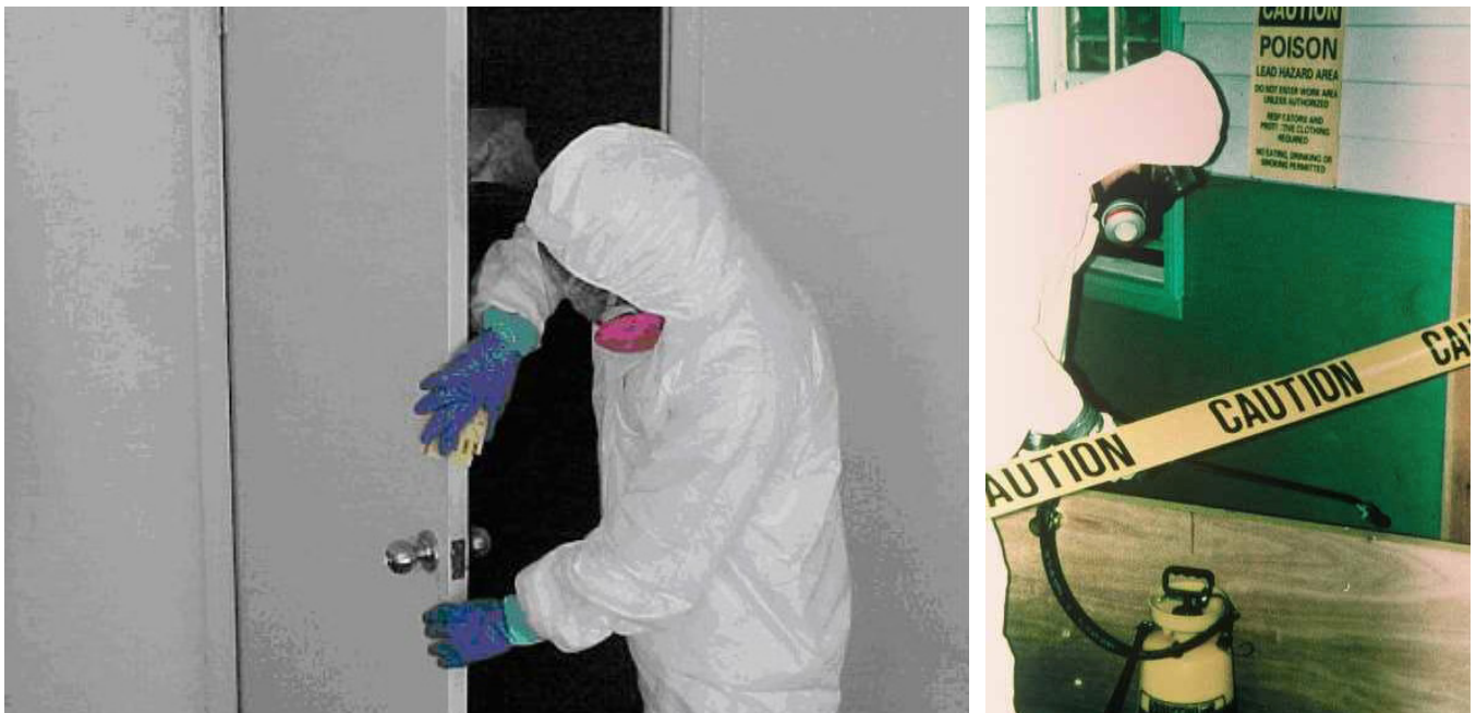
FIGURE 11.15 Stabilizing paint on doors: Wet planing (left) and wet sanding (right) deteriorated paint can create significant amounts of dust.
