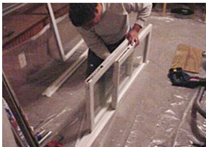
Figure 11.13 Fit sashes into jamb liners.
