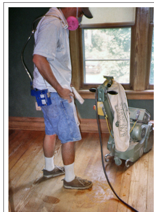
FIGURE 4.1 Sanding wooden floors can generate significant amounts of dust.
