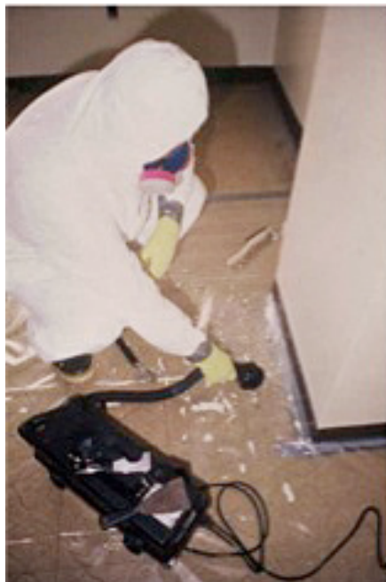
FIGURE 14.8 Vacuuming the floor containment.
