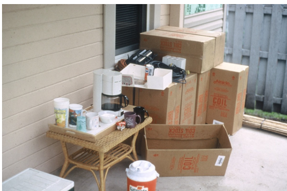
FIGURE 8.7 Placing coffee station in the work area is an unsafe work practice.
