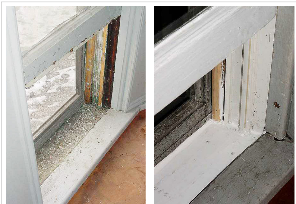
FIGURE 11.3 Window before and after friction treatment.
