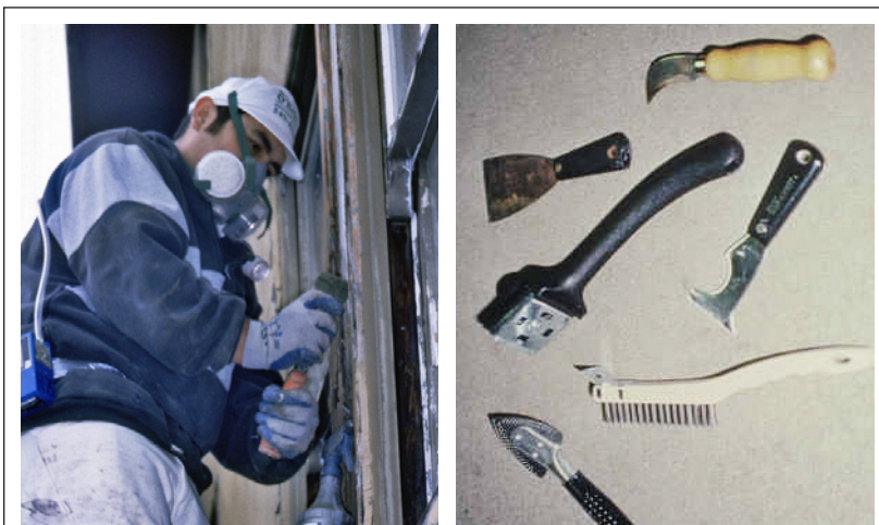
FIGURE 12.16 Wet scraping (left) FIGURE 12.17 Scraping tools (right).
