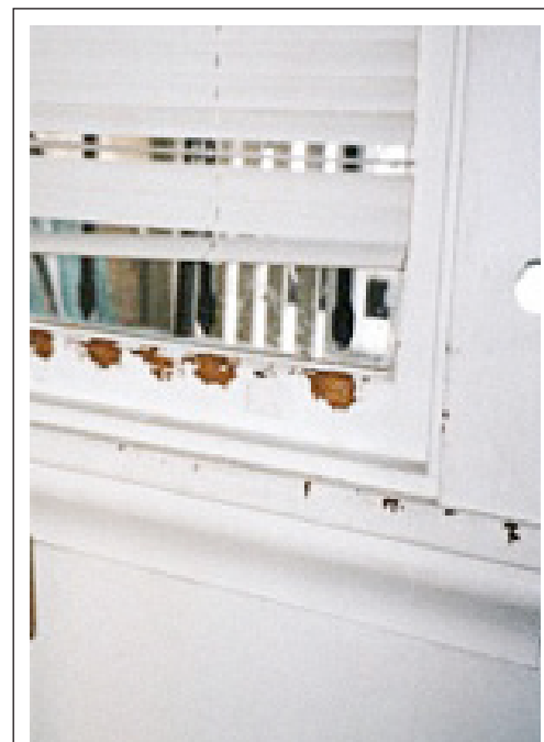
FIGURE 5.8 Chewable surface: teeth marks on window sill.
