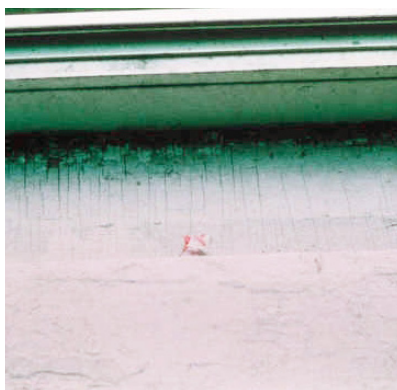
FIGURE 5.4b Alligatoring paint
