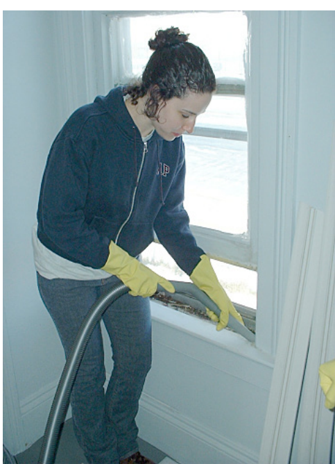
FIGURE 8.17 Pre-cleaning window with HEPA vacuum.
